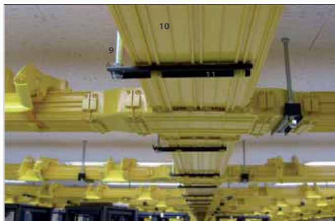
2. Example of OptiWay installation from the ceiling
